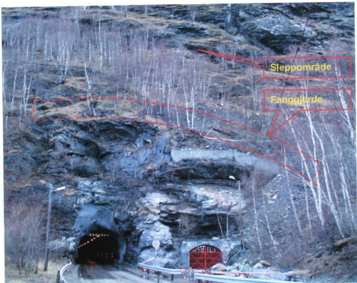
1: Fv. 303, Seimsdaltunnelen aust, km 2,510, 13-01-2005
